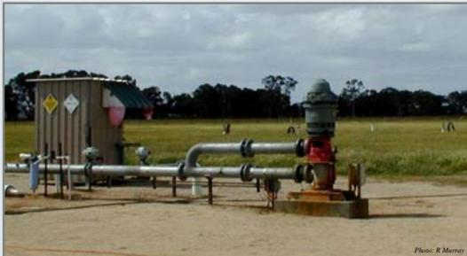
Treated waste water is injected into a confined limestone (non-karstic) and sand aquifer and later used for irrigation
