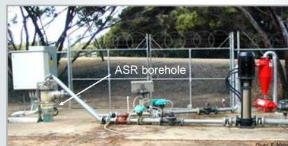
ASR borehole, Adelaide, Australia. Urban runoff is diverted into a constructed wetland for treatment and then injected into a limestone aquifer.
