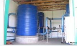
Pre-treatment: City's drinking water further treated with Granular Activated Carbon & chlorination
