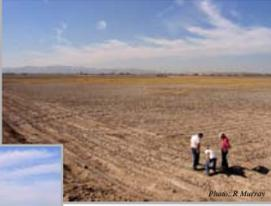
Infiltration basin, Phoenix, Arizona, USA. Water from the Colorado River is diverted into a number of shallow infiltration basins.
